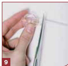
9 Line up with old tubing and cut...
